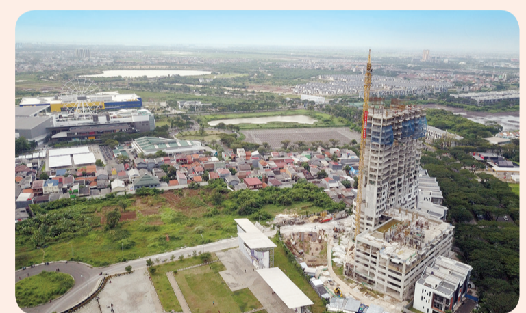
Progress Cleon Park Apartment.
